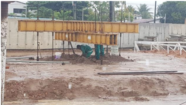
Figure 6 – System of reaction beams.
